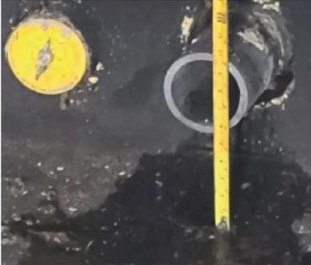
R The outlet end of the overflow has been fitted with an angle-flap valve, see photo below. The outlet end of the drain is operated by a valve and has no potential for rodents or debris to enter the system.
