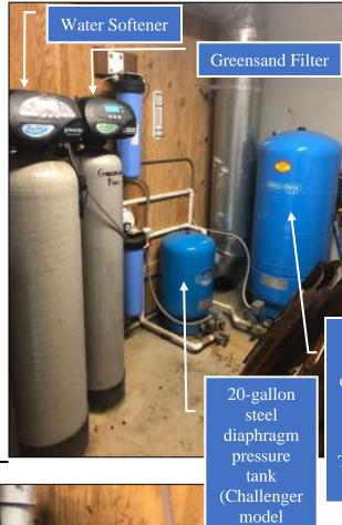
81-gallon steel diaphragm pressure tank (Well-X-Trol model wx255)
