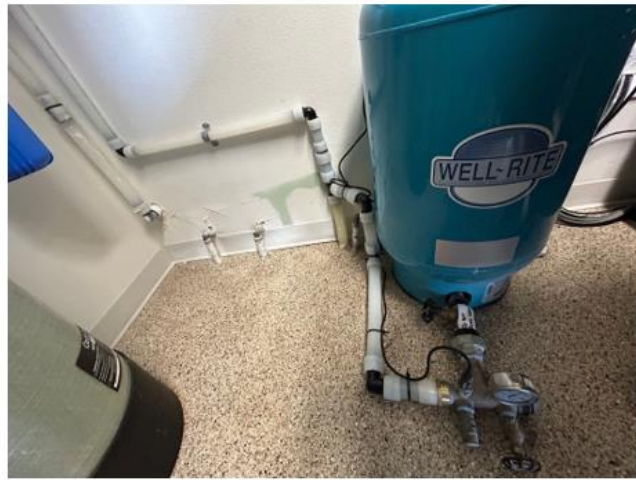
Water enters building to pressure tank. Make: Well-rite Model: WR60R
