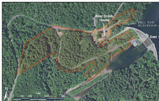
Figure 6b: Bull Run Reservoir 1 Bear Creek House Area (Location # 6)
